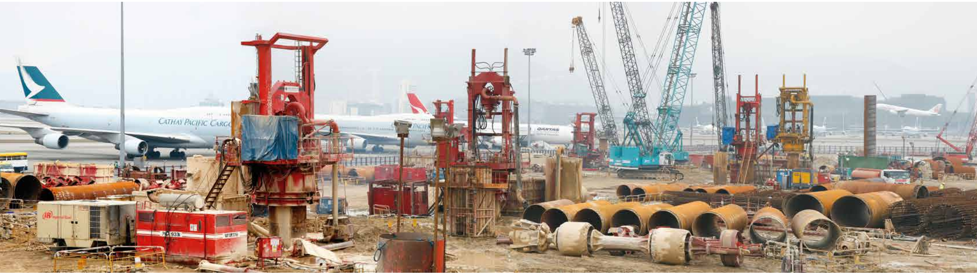
Terminal Midfield | Hong Kong BACHY SOLETANCHE GROUP LIMITED
