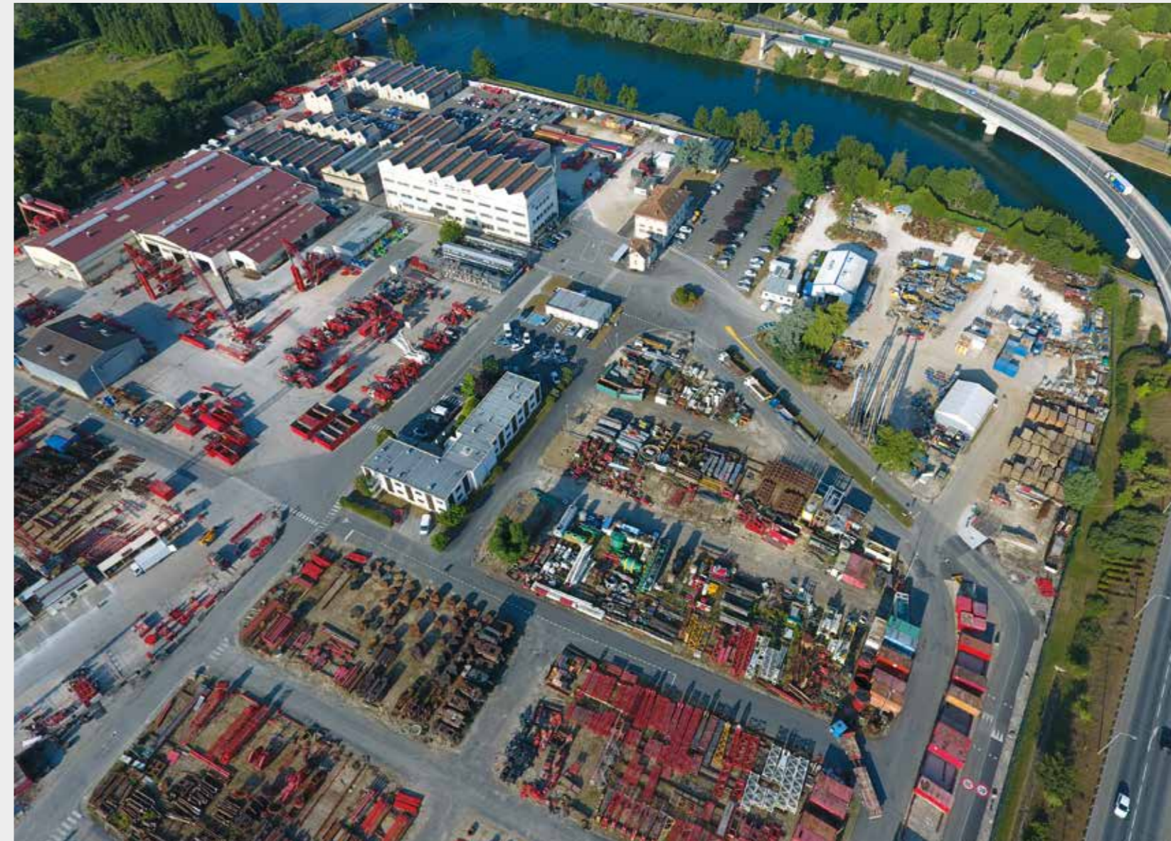
Plant yard and fabrication and maintenance facility | France
