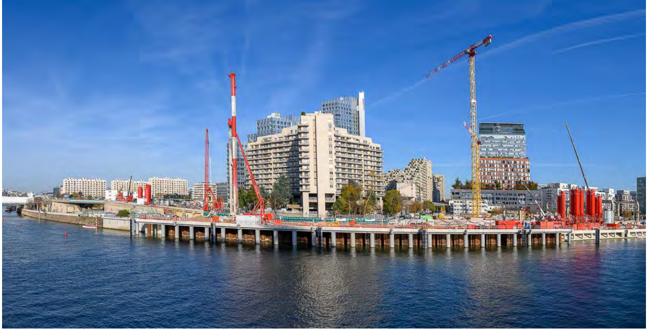
Fig. 3 – Pile boring machine making deep soil mixing columns ©C.Helsly
