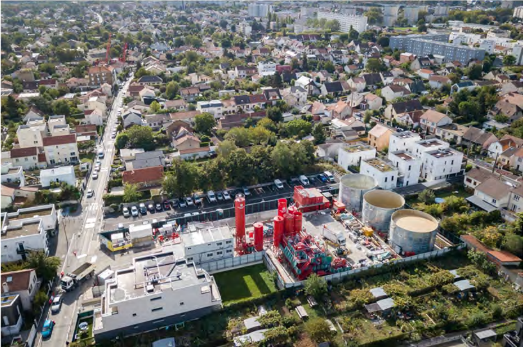
Fig 3 : Overview of the slurry wall installation located 360 m downstream from the site - © Cédric Helsly
