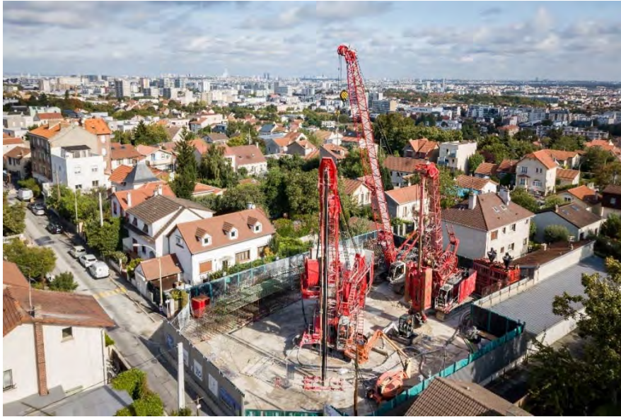
Fig 6 : D-wall excavation with hydraulic grab and Hydrofraise® - © Cédric Helsly
